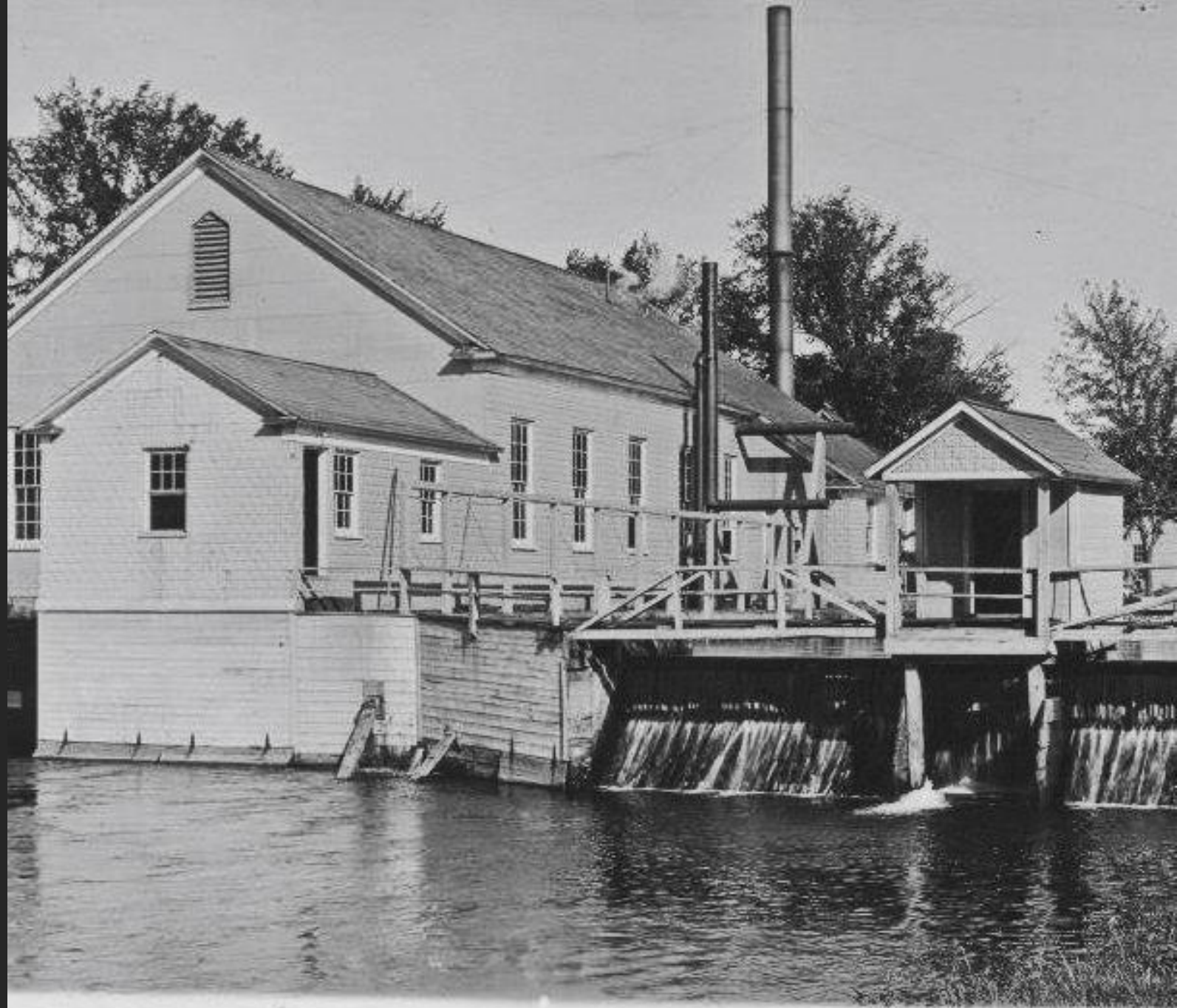
50—Electric Light Power House, Sidney, N. Y.
